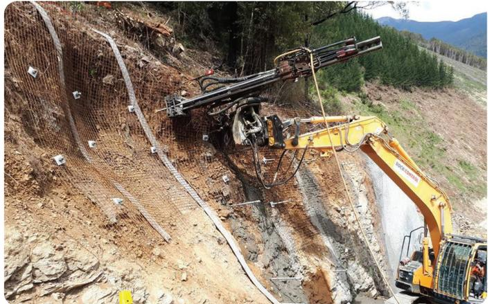
Constructing permanent stabilisation to colluvium deposit on the right hand side
