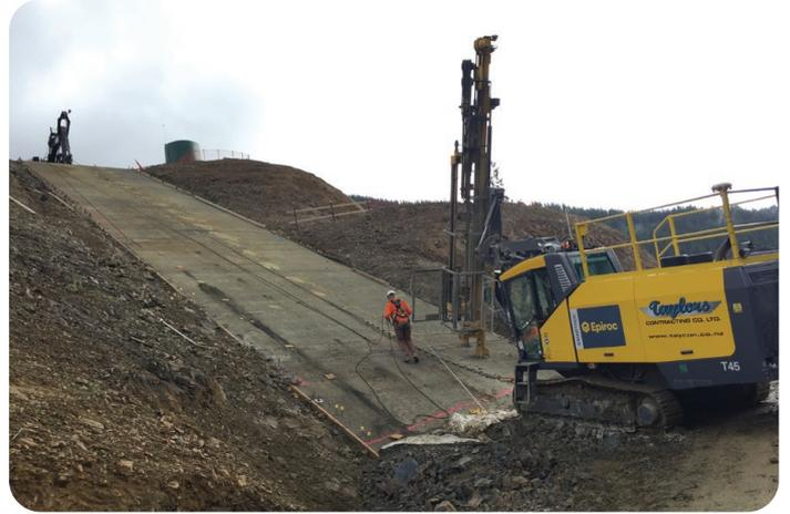
Drilling anchors for the left hand plinth
