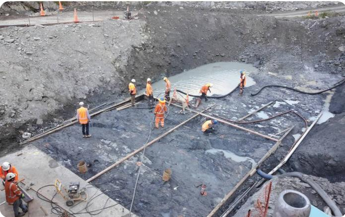
Preparing the culvert foundation - note void to be filled
