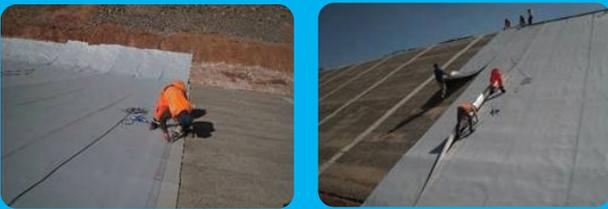
Most recently used in New Zealand on the Tekapo Canal, the membrane is a geocomposite material comprising of a plasticised polyvinyl chloride (PVC-P) geomembrane
