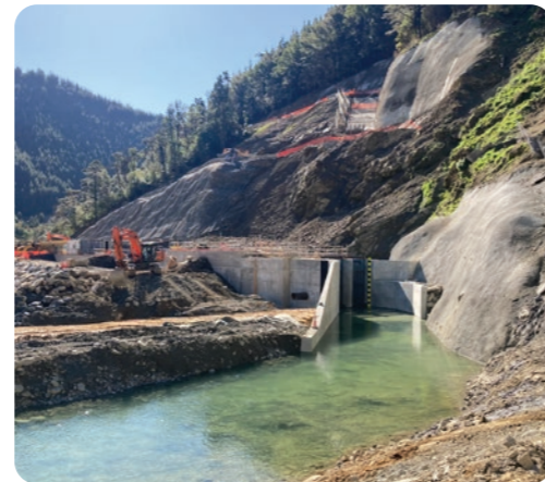
The river was diverted through the culvert on 2 September.
