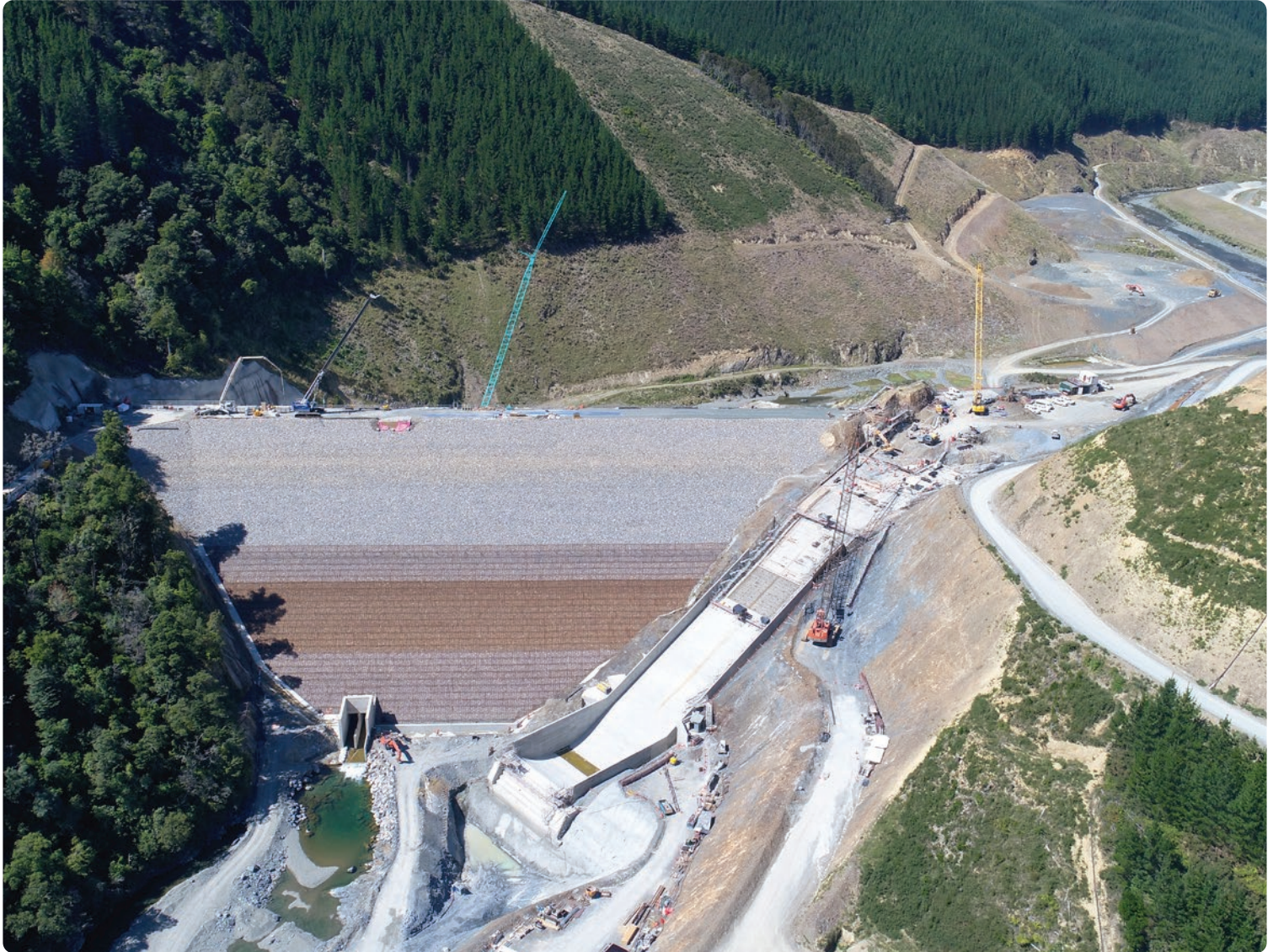
The Waimea Community Dam more than 70% complete. March 2022.
