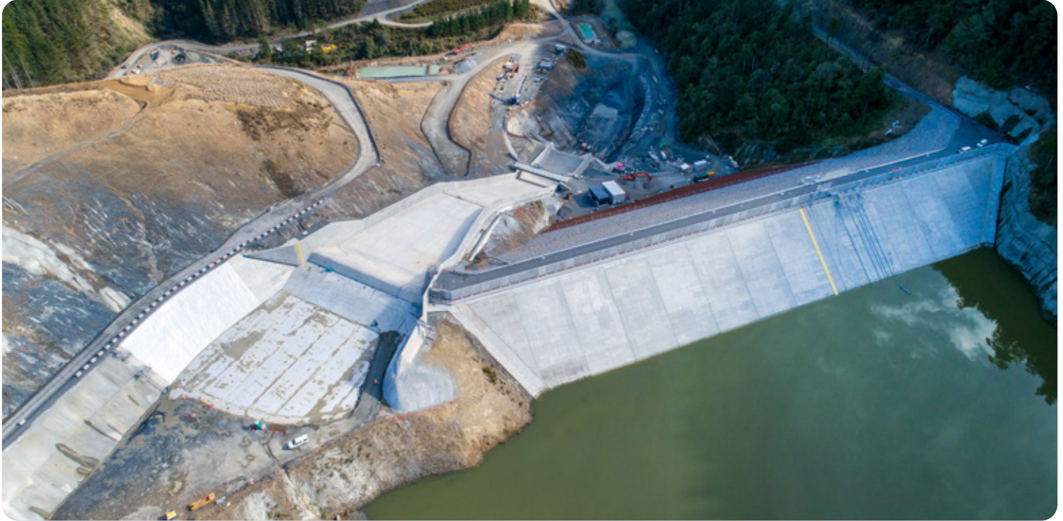
Dam and spillway complete. Reservoir filling in stages, September 2023.
