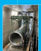
The two intake pipes enter the UPSTREAM VALVE CHAMBER, where water quality is achieved by mixing the flows from the two pipes using butterfly valves.
