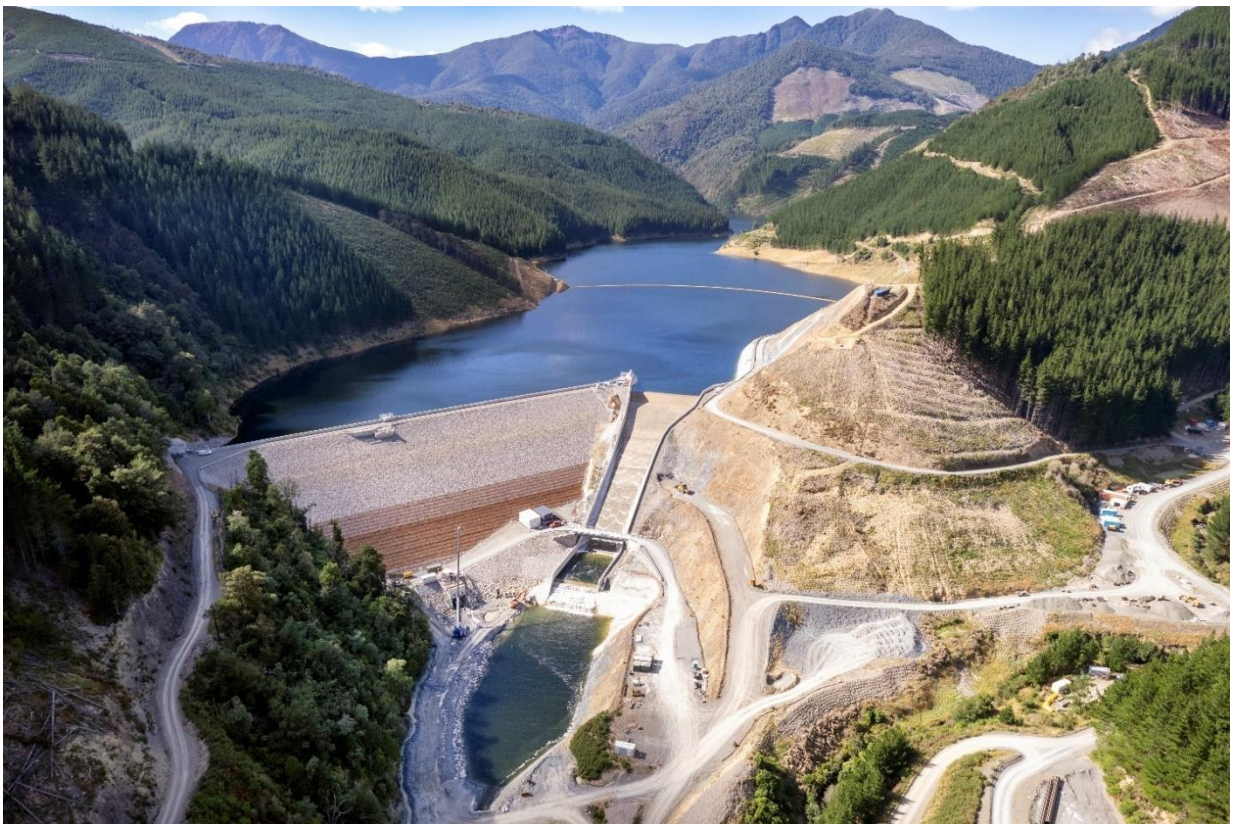
Figure 1 First week after reservoir filled and spillway in use – 30 Jan 2024
