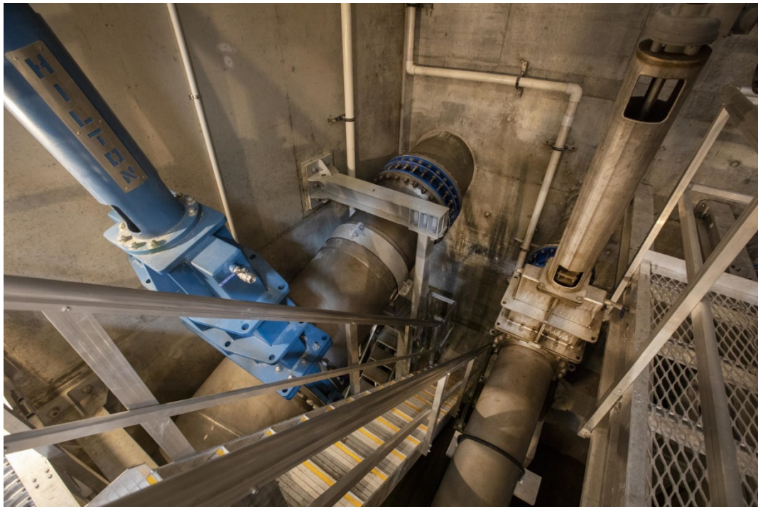
Figure 5: Access inside the valve chamber is completed, August 2024.
