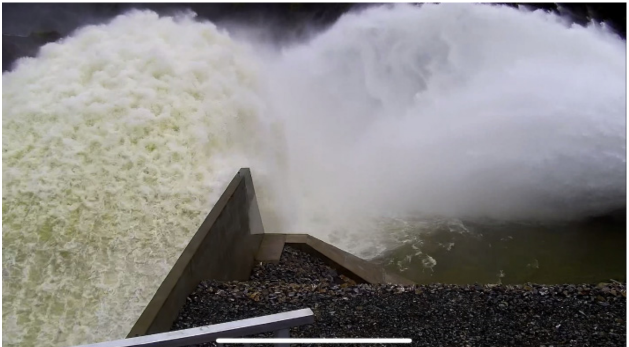
Figure 2: 136m 3 /s of water landing in the plunge pool on 3 October 2024.
