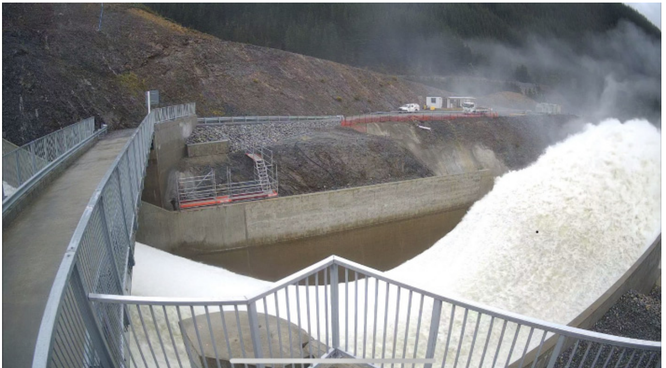
Figure 6: 136m 3 /s of water on 3 October 2024 provided the largest load to the spillway to date.
