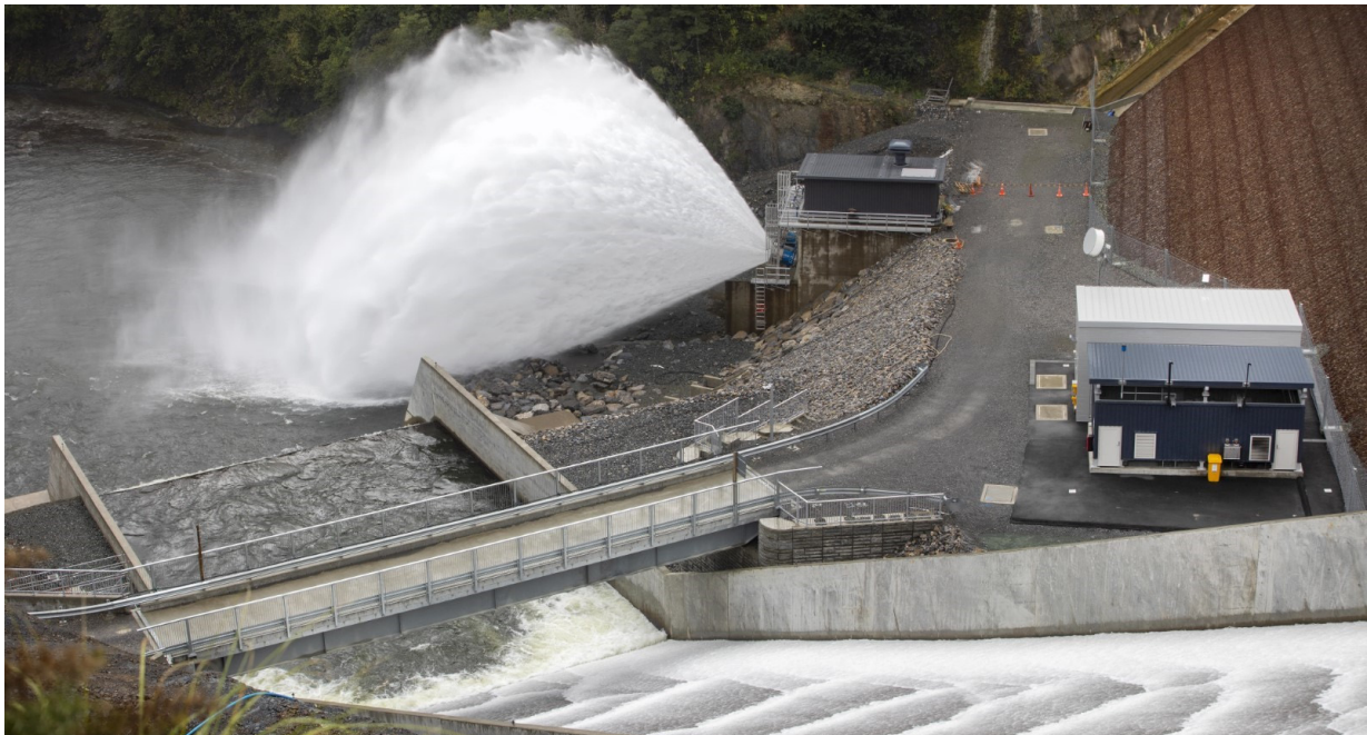
Figure 3: Waimea Community Dam was deemed fully operational during the period.
