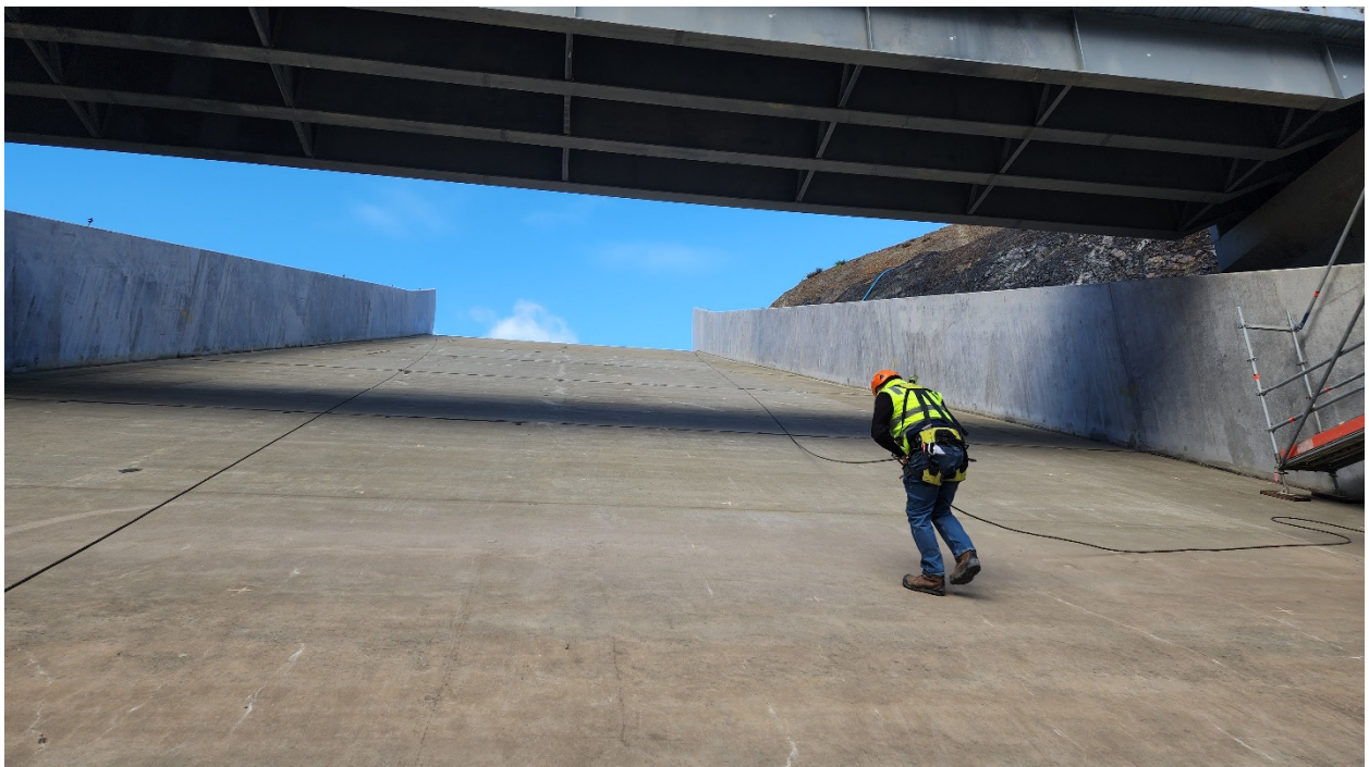
Figure 4: Inspection of the spillway chute.
