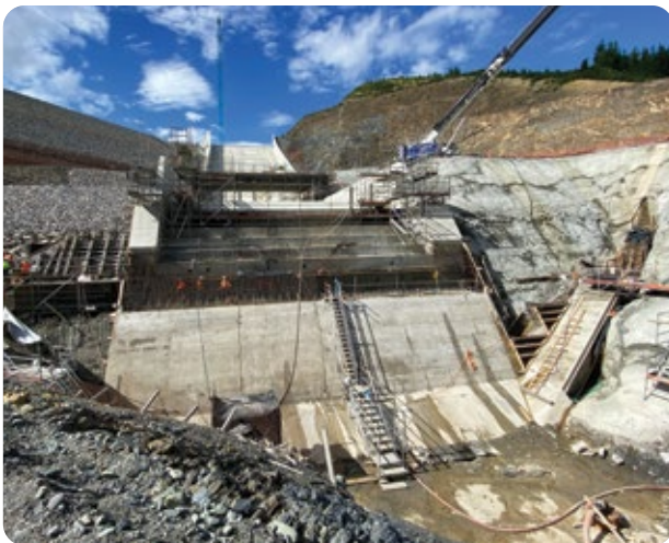
A nine metre cut-off wall below the flip bucket.
