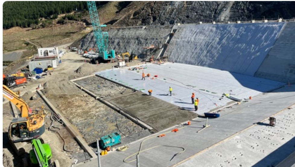
Carpi waterproof liner being placed on the spillway approach, April 2023.
