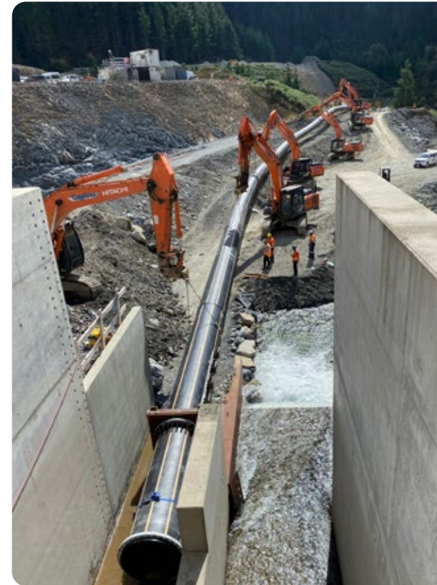
Installing temporary river diversion HDPE pipe in left culvert.
