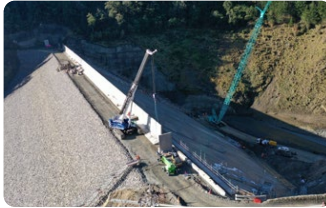
Installation of the parapet wall on the dam's crest, June 2022.
