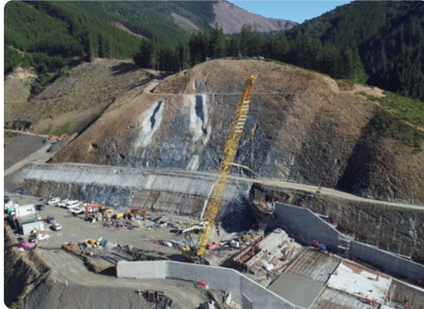
A view of the fractured true LHS with shear zones above the spillway.
