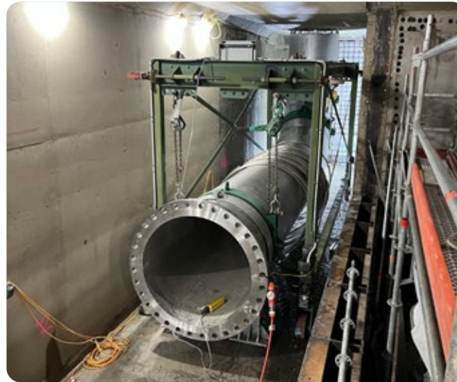
Installing lobster back bend pipe.
