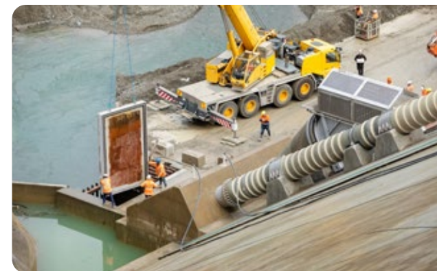
The second stoplog installed to permanently close the river diversion, 26 May 2023.
