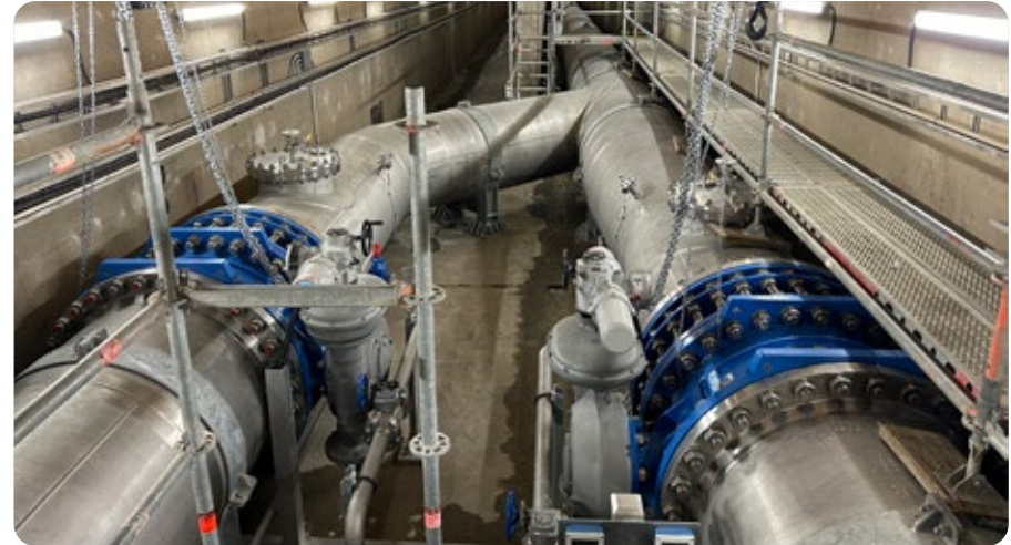
Intake pipes and PIVs.
