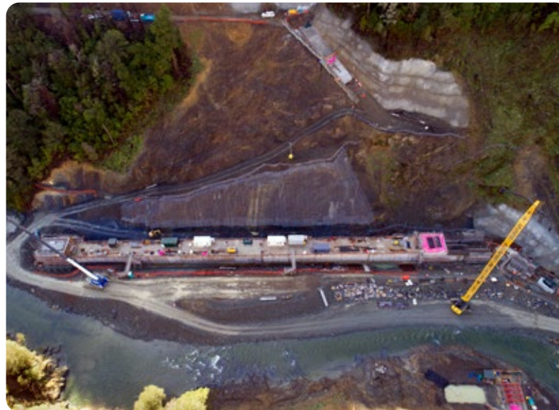
The culvert was constructed of 4,500m 3 of concrete and 815 tonnes of steel.
