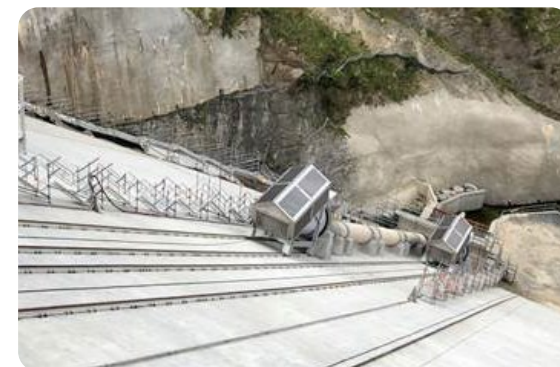
Intake screens and pipes on the dam face.
