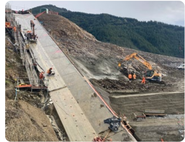
The plinth being constructed, 2020.
