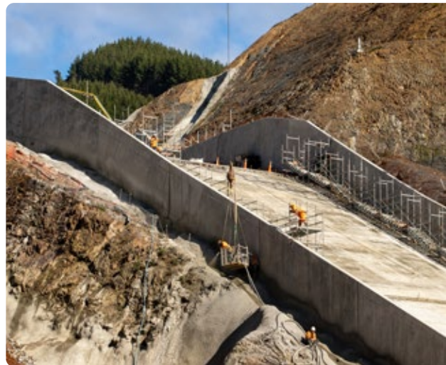
Free-standing cantilevered spillway walls above the steep topography.
