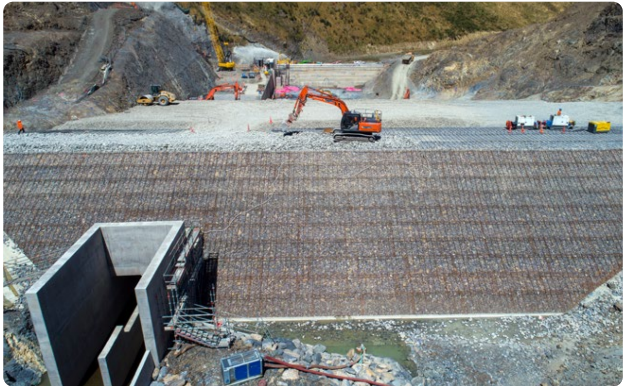
The completed rockfill face protects the embankment during construction.
