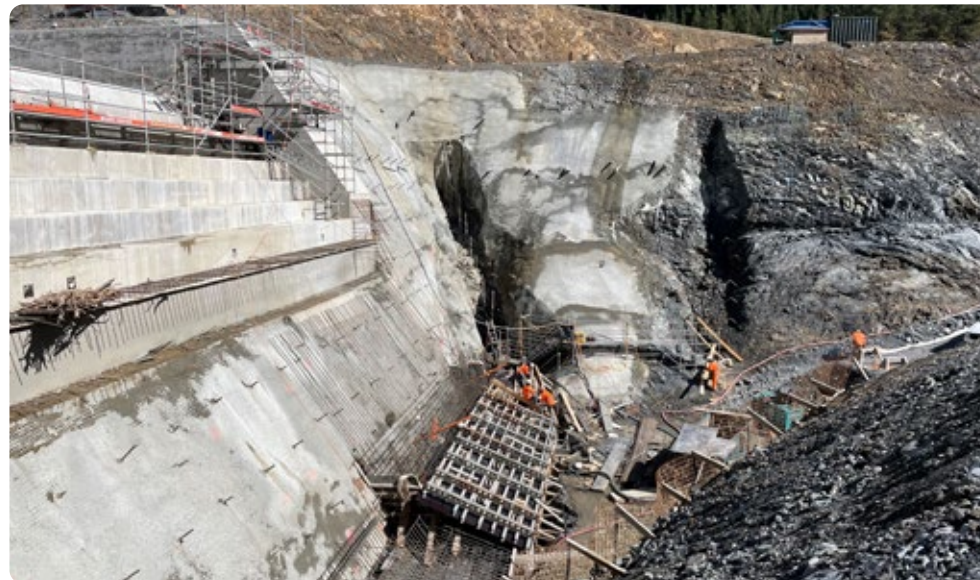
Constructing the cut-off wall at base of flip bucket and plunge pool shotcreting.
