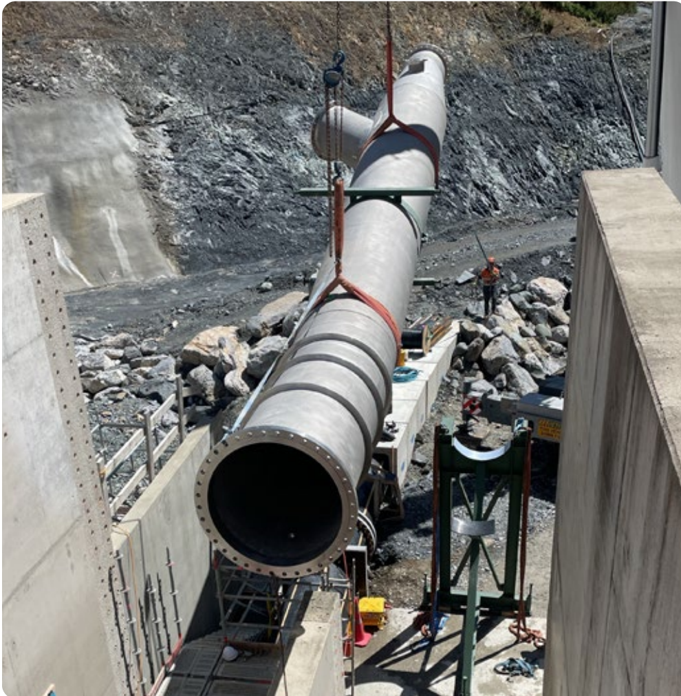
Fifteen-degree bend pipe being lifted into position at the culvert outlet chamber.
