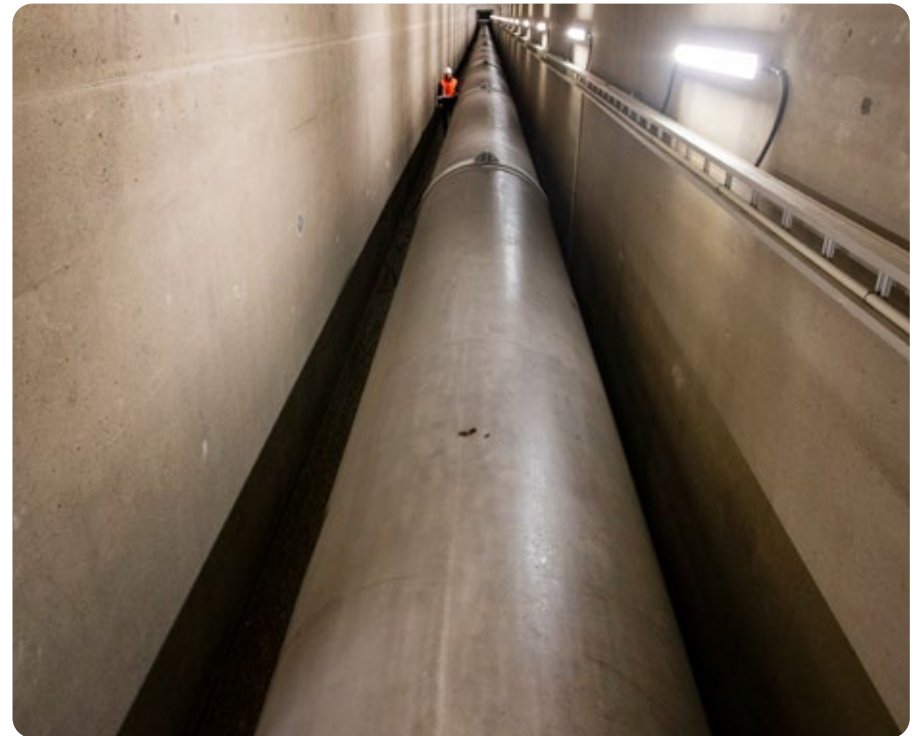
1.4 metre diameter stainless steel pipe in the right culvert.
