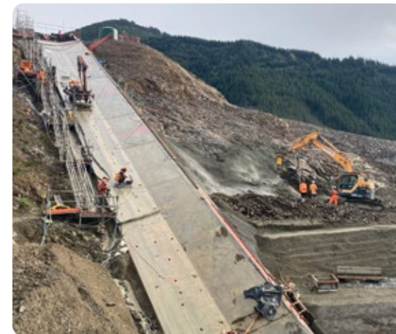
Grout curtain being drilled through true left plinth slabs.
