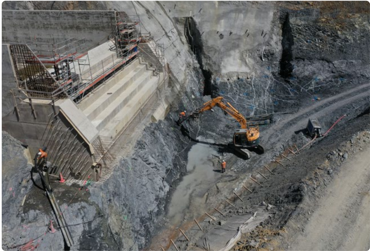
Extensive remedial work required at the base of the spillway and plunge pool.
