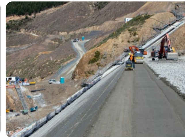
Flow-limiting zone on left and chimney drain on right.
