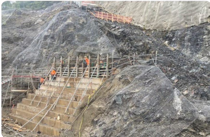
Stabilising structures under the RHS plinth.
