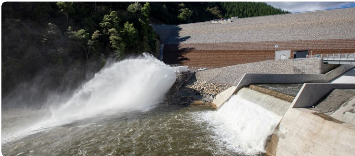
The two large fixed cone valves tested, commissioned and ready for operations, April 2024.
