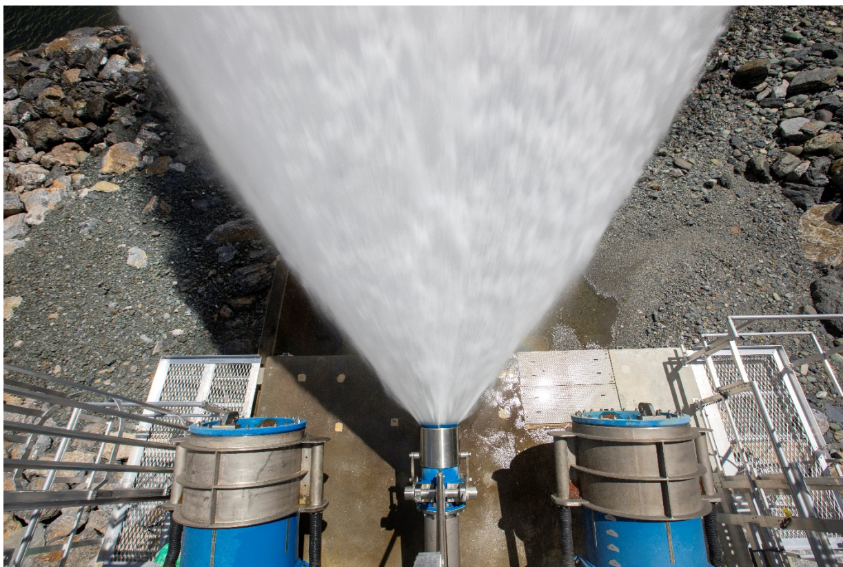
Figure 1 The three dispersing cone valves, one in action
