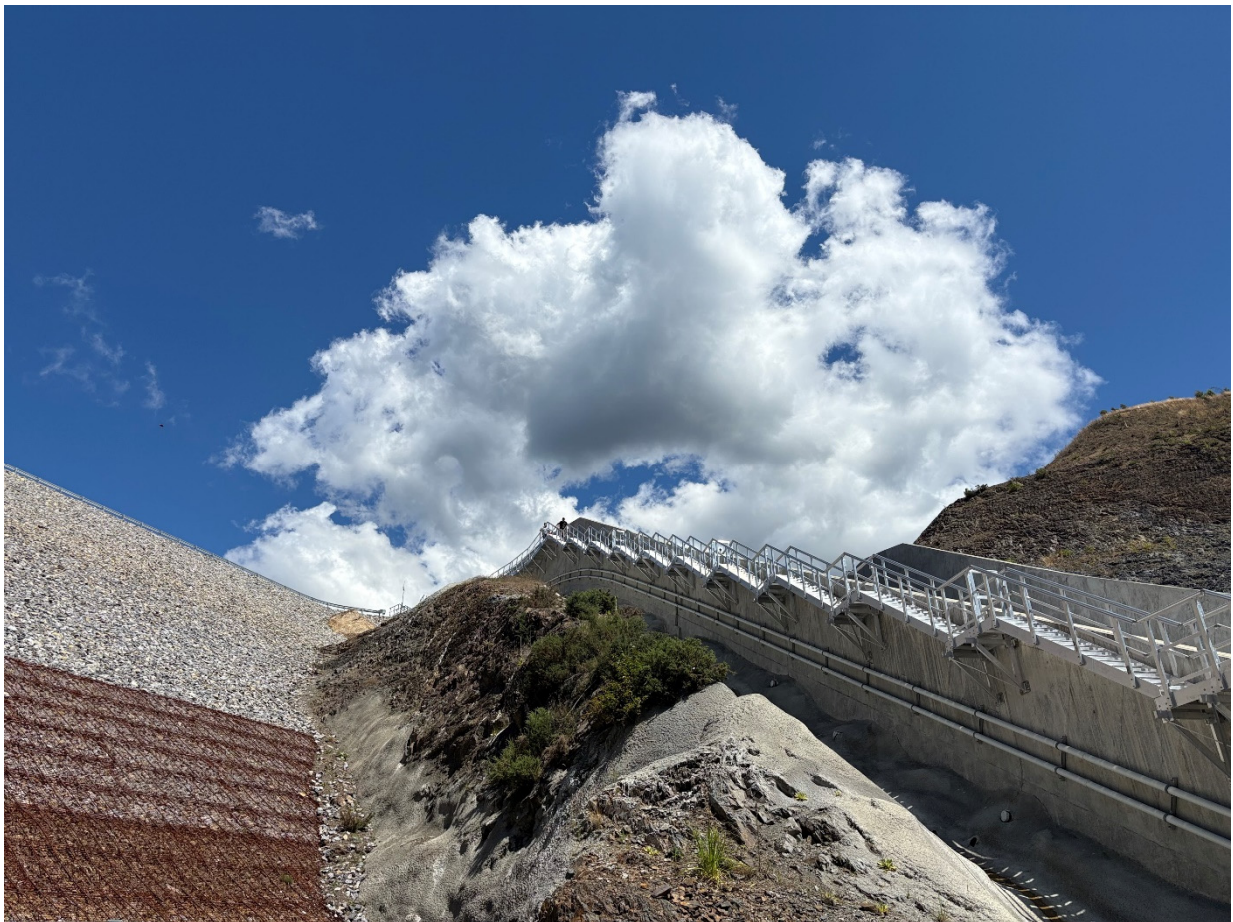
Figure 1 Looking up at the spillway stairs
