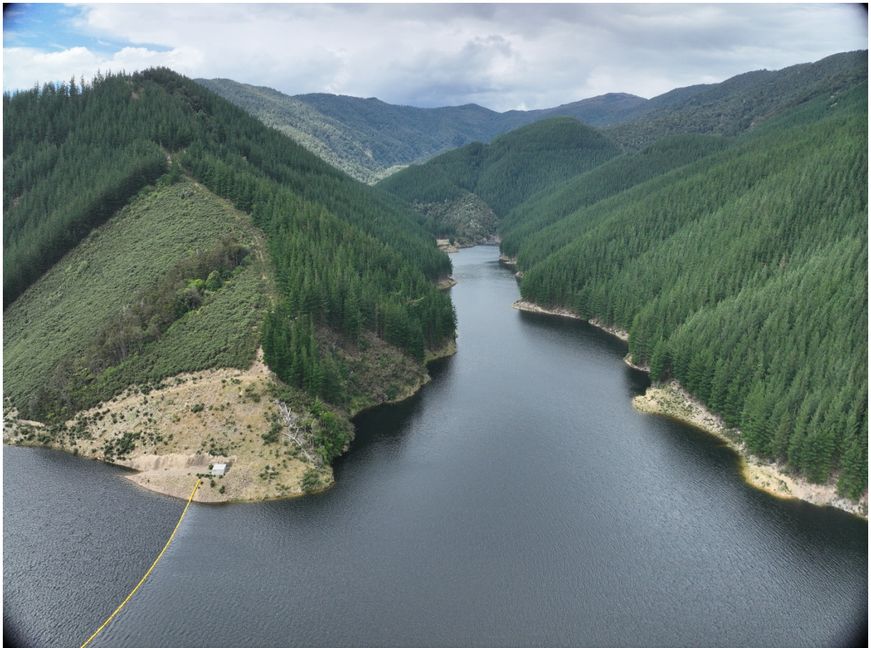
Figure 3 The Waterfall Creek section of the reservoir, Te Kurawai o Pūhanga
