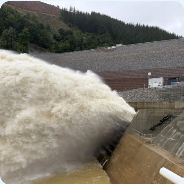
The flipbucket dispersing the water’s energy from the rapid flow down the spillway, 2 June 2026.
